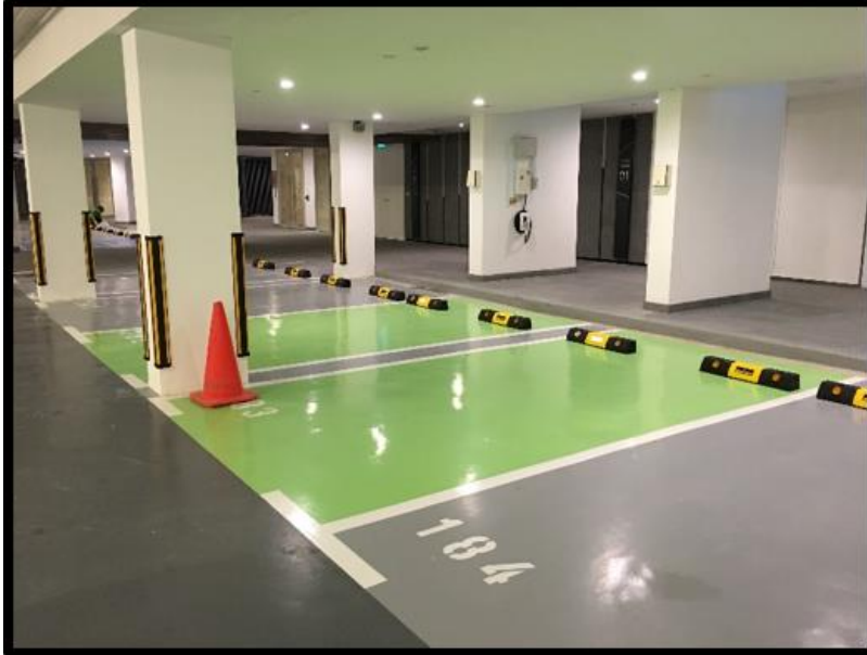
Fig. 4.6b Demarcation of parking lots using different colour tone and serially numbered
