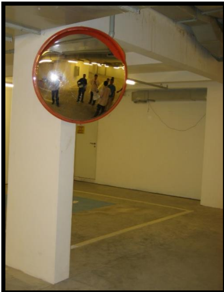
Fig 4.9c Convex mirror can be provided at corners and blind spot areas to provide better visibility for motorists and pedestrian.
