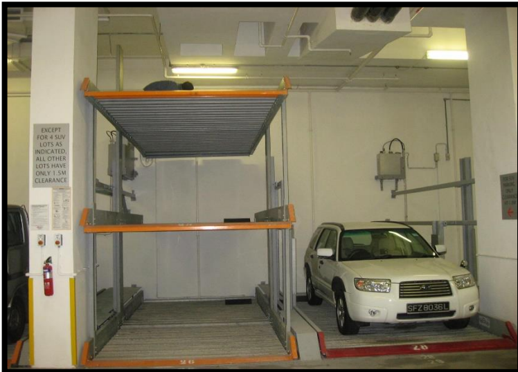
Fig 3.1c Stack-type vertical system
