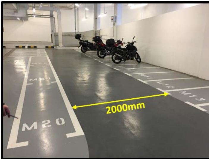
Fig 2.3.1c Parking aisle for motor-cycle
