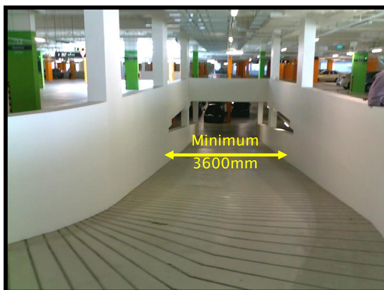
Fig 2.1.3d Example of a single, straight lane
