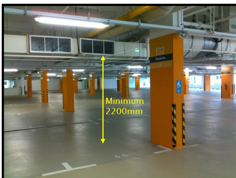
Fig 2.1.5b Example of minimum headroom clearance
