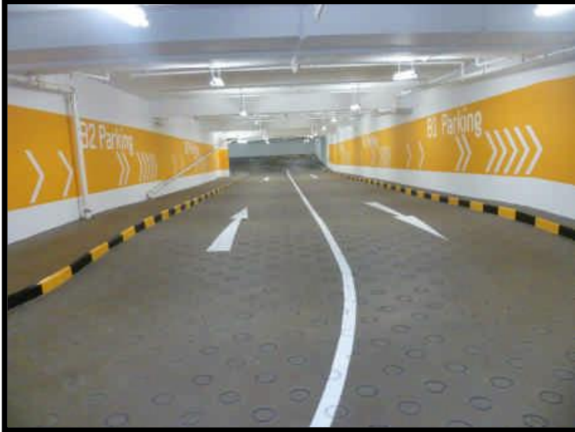
Fig. 4.9b Use of traffic markings, painted kerbs along narrow driveway
