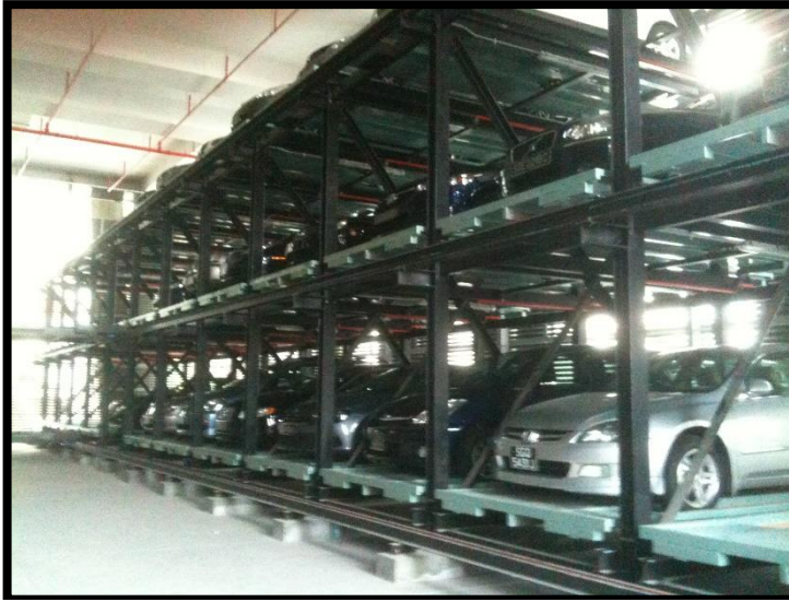
Fig 3.1b Car storage space of a fully-automated system
