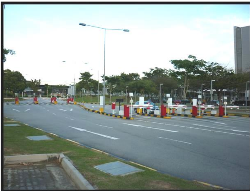
Fig. 4.13b Example of multiple entry/exit points and long queuing space
