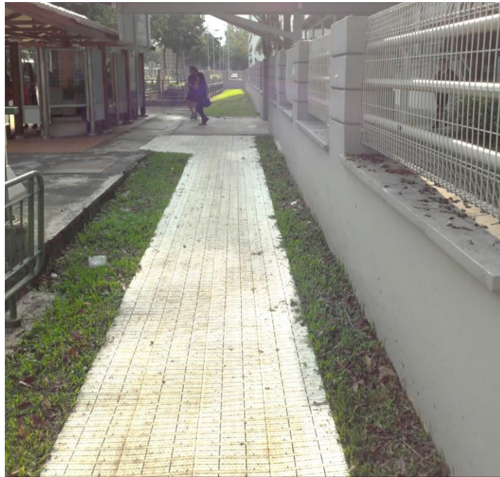
Picture 1 – Portable Protective Flooring implemented by Shincon Industrial Pte Ltd
