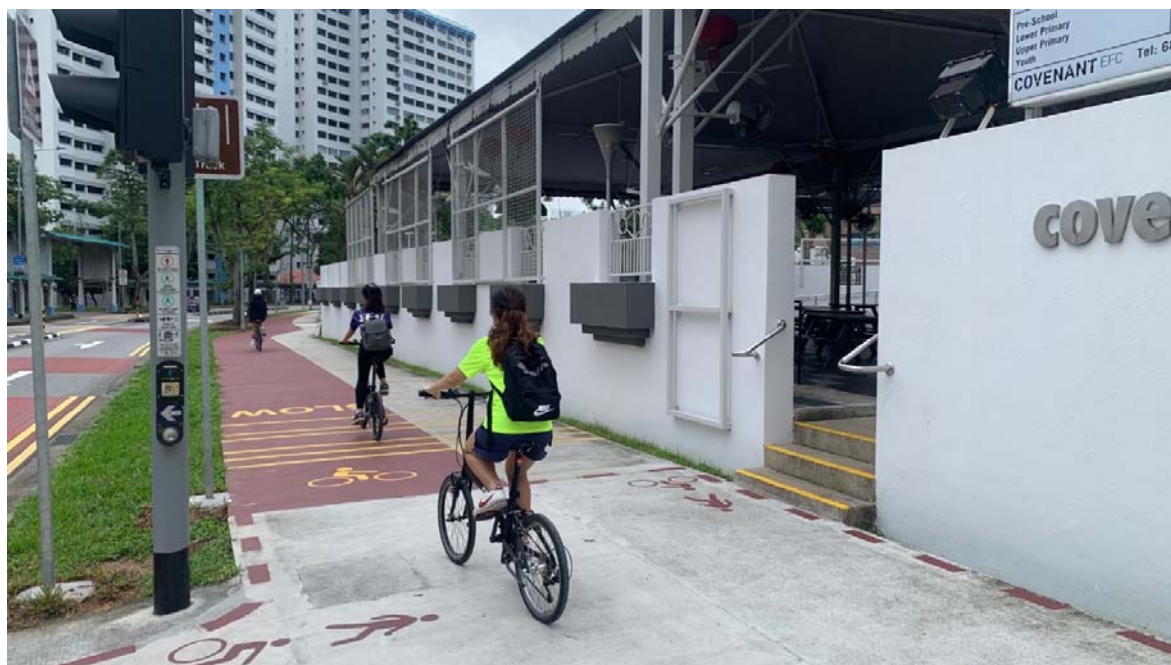
Widened path with repurposed road space at Jelapang Road
