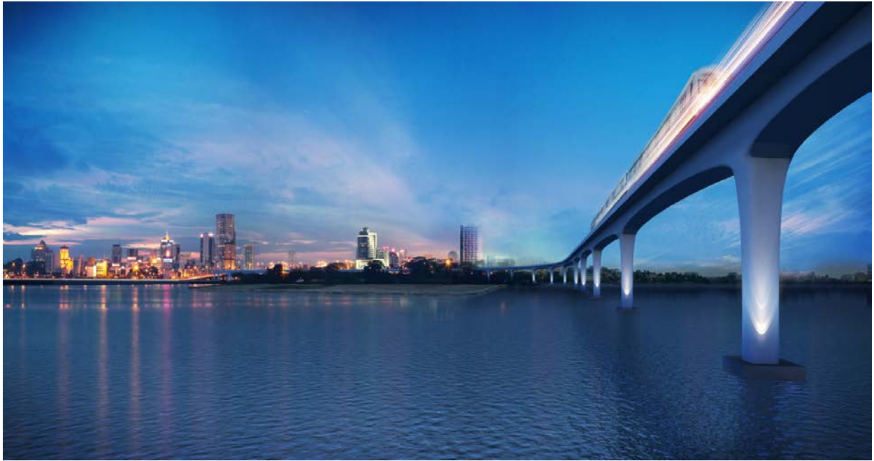
RTS Link viaduct
