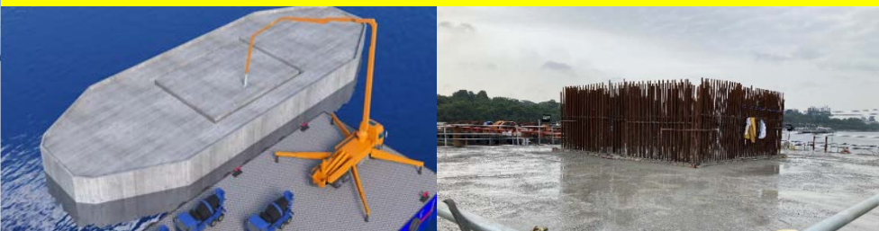
5. Concrete Casting of Pilecap
