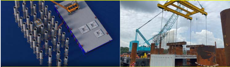
2. Installation of Steel Side Formwork
