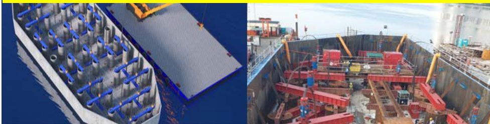
4. Hacking of pilehead & rebar works
