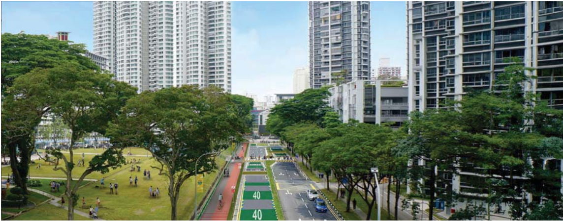
Street signs, green road surface markings and road humps to remind drivers to slow down
