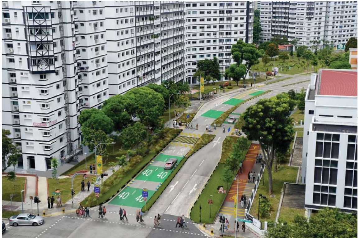
Street signs and green road surface markings when entering and driving along Friendly Streets to remind drivers to slow down
