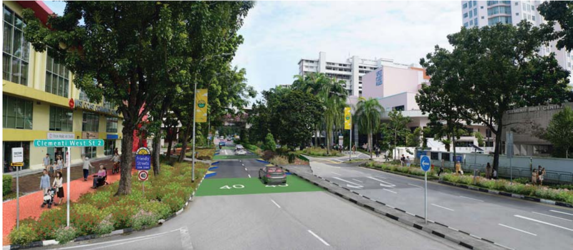
Street signs and green road surface markings when entering and driving along Friendly Streets to remind drivers to slow down
