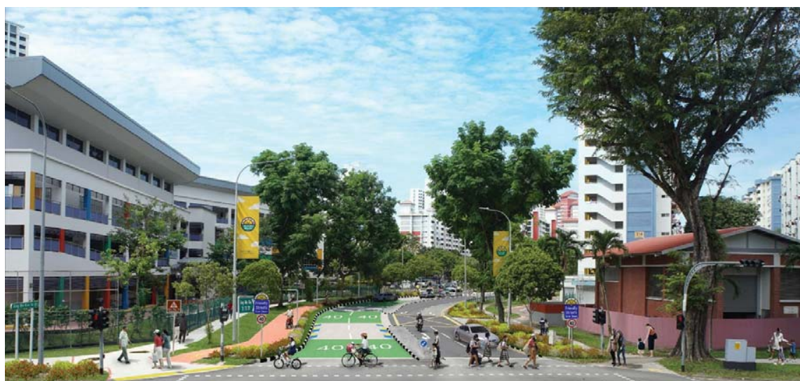
Street signs and green road surface markings when entering and driving along Friendly Streets to remind drivers to slow down
