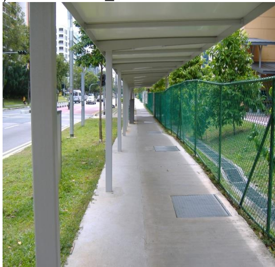
Type 1PF - Single pole flat roof
