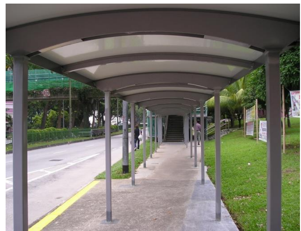
Type 2PC - Double pole curve roof
