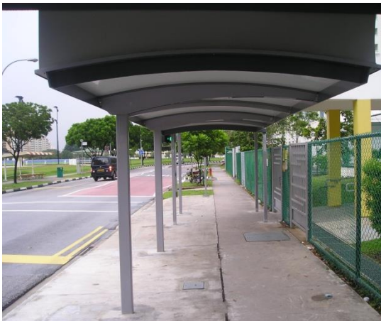
Type 1PC - Single pole curve roof
