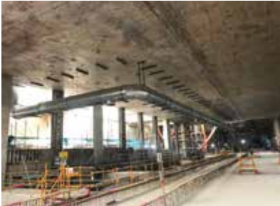
Provision of ventilation fan and duct
