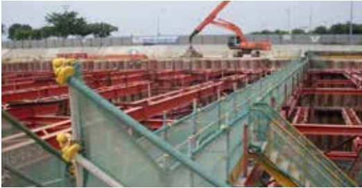
Proper walkways provided along struts
