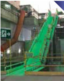
Walkways were provided to ease evacuation in case of emergencies
