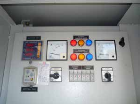
Distribution board with Residual Current Circuit Breaker (RCCB) and other safety devices
