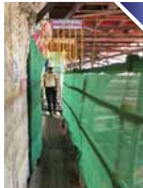
Walkways were provided to ease evacuation in case of emergencies
