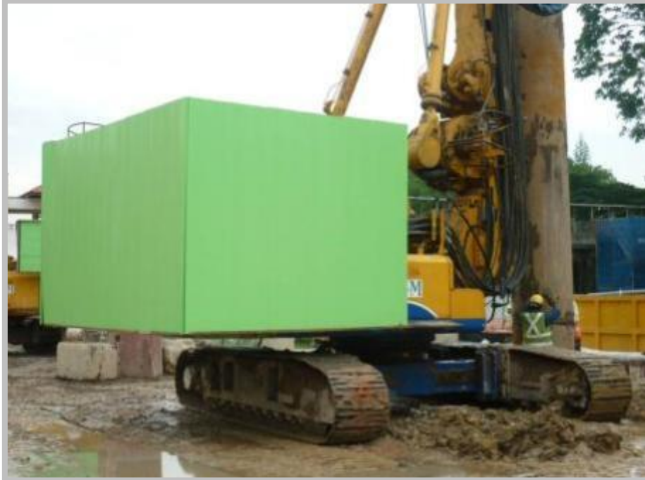
Noise enclosure on boring rigs
