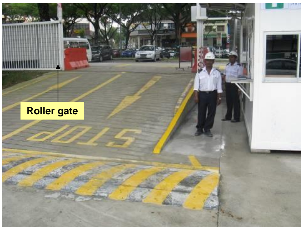
Roller gate at the entrance has an advantage over hinged gate as it eliminates the accidental swinging of gate that can result in hitting man or vehicle
