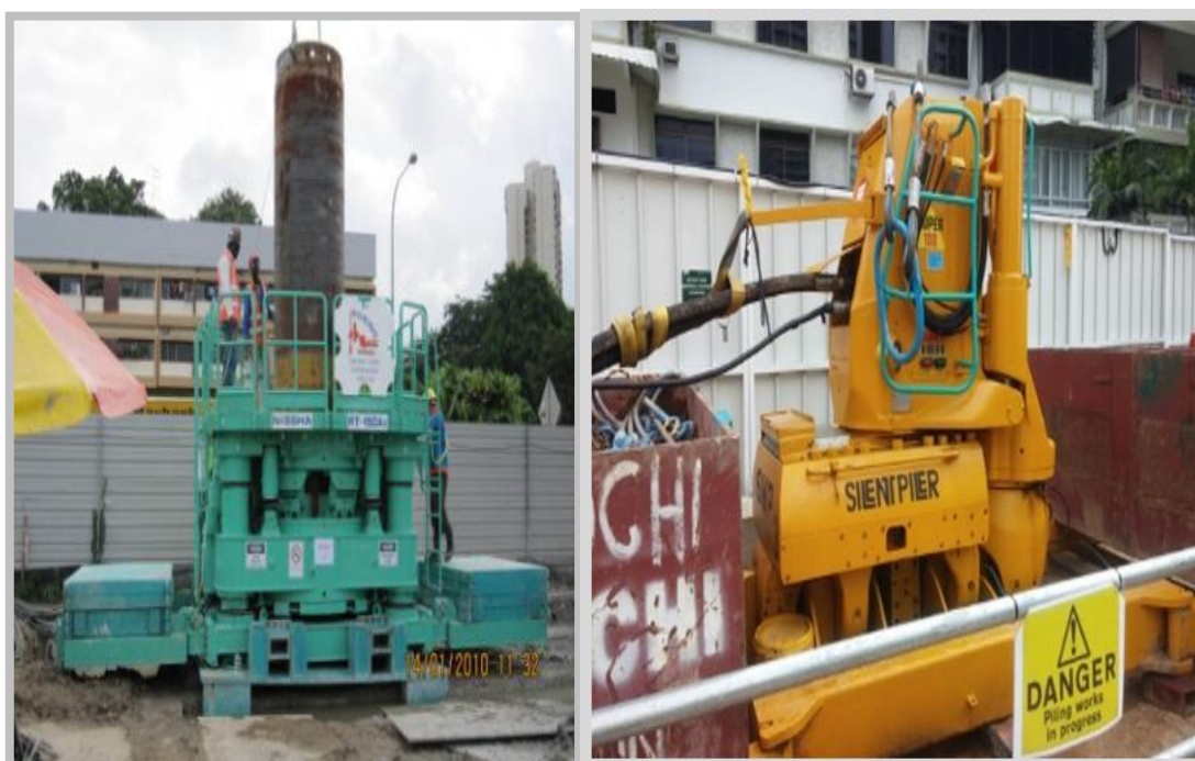
Use of silent-piling machine (for suitable soil conditions)
