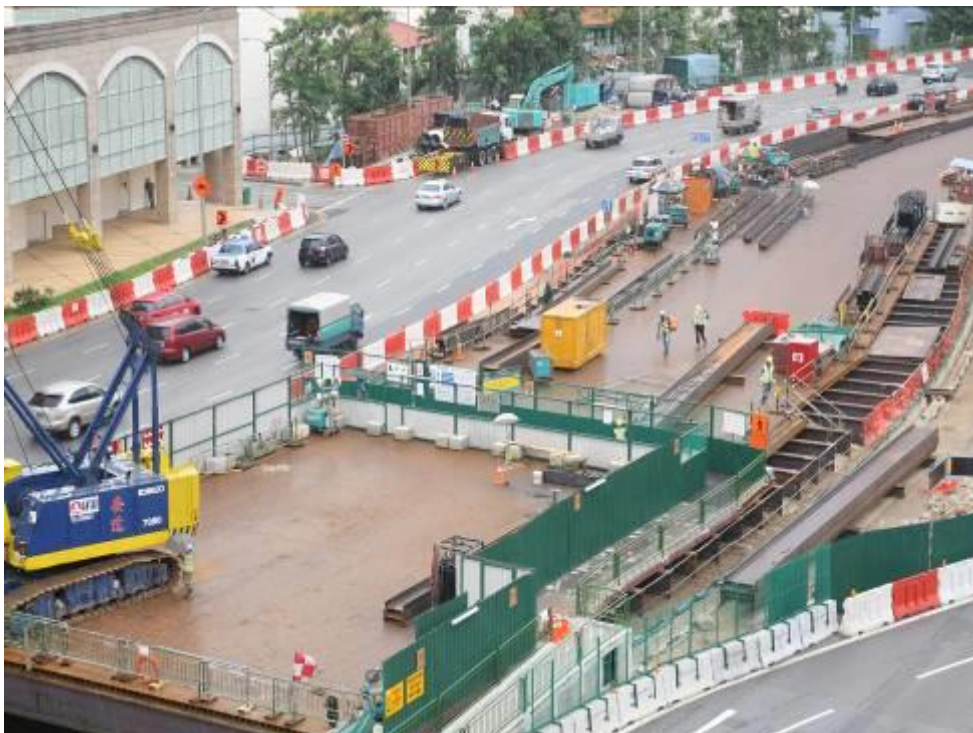
Good housekeeping around worksite
