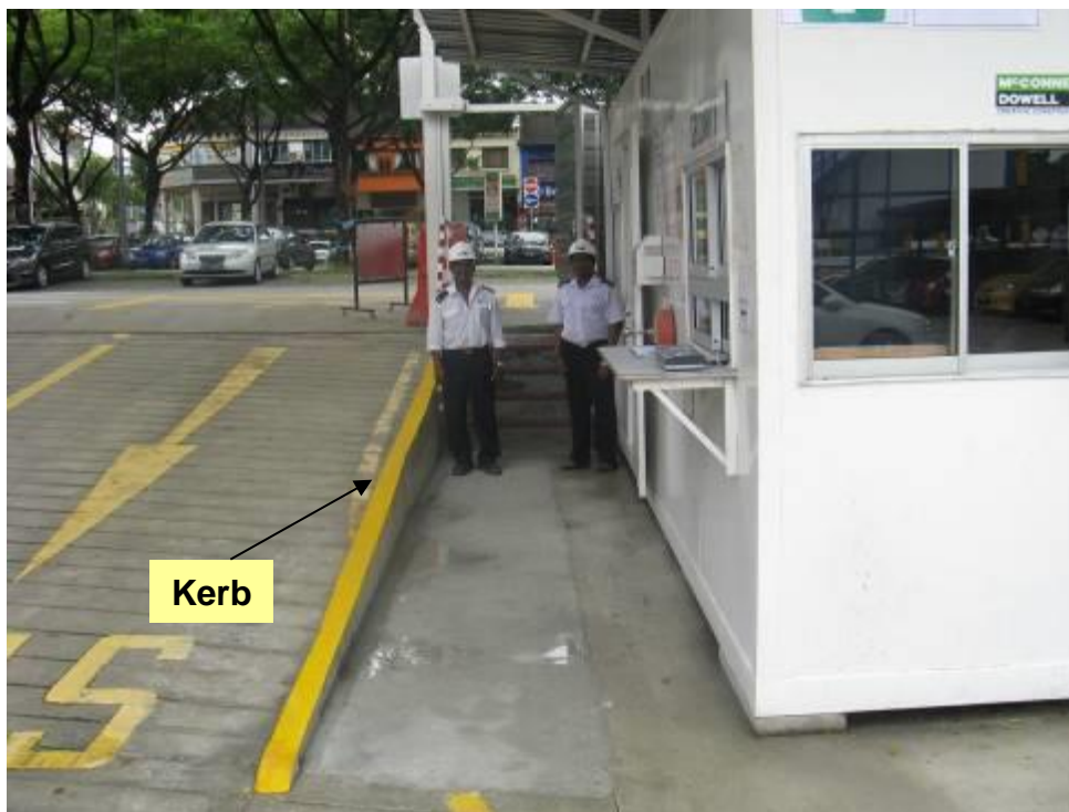
Security pass exchange area separated from vehicle access to prevent vehicles driving too near and injuring workers reporting at the security post
