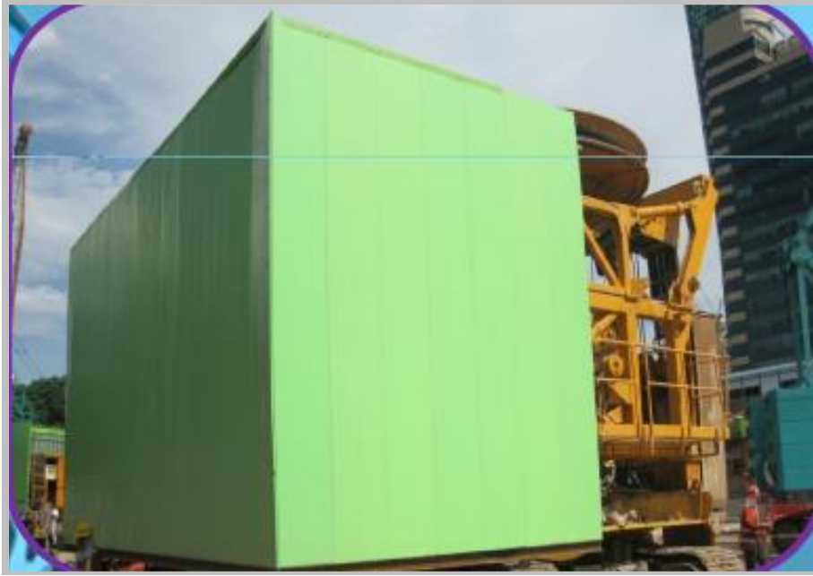
Noise enclosure on D-wall cutter machine
