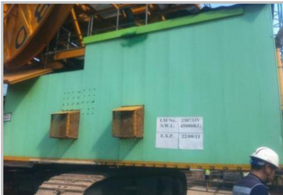
Noise enclosure on D-wall cutter for ventilation fans
