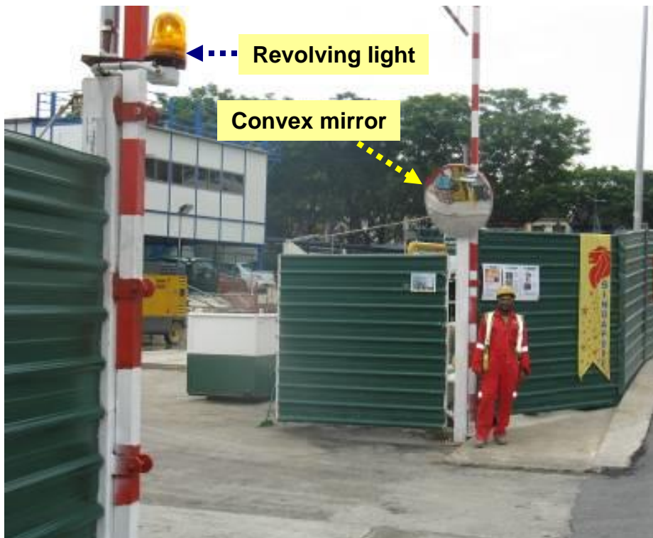
Site entrance equipped with revolving light and convex mirror to enhance pedestrian safety. Full-time banksman deployed to guide vehicles exiting the worksite
