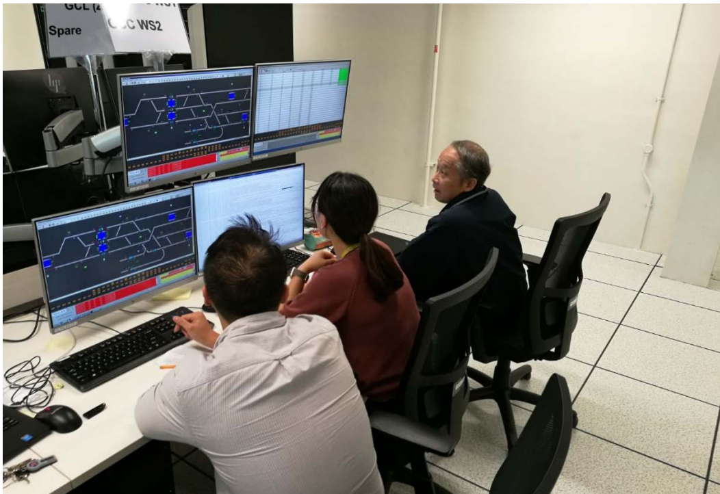
Photo 4: The software of new signalling system was tested at the signalling simulation facility before deployment on the main track.
