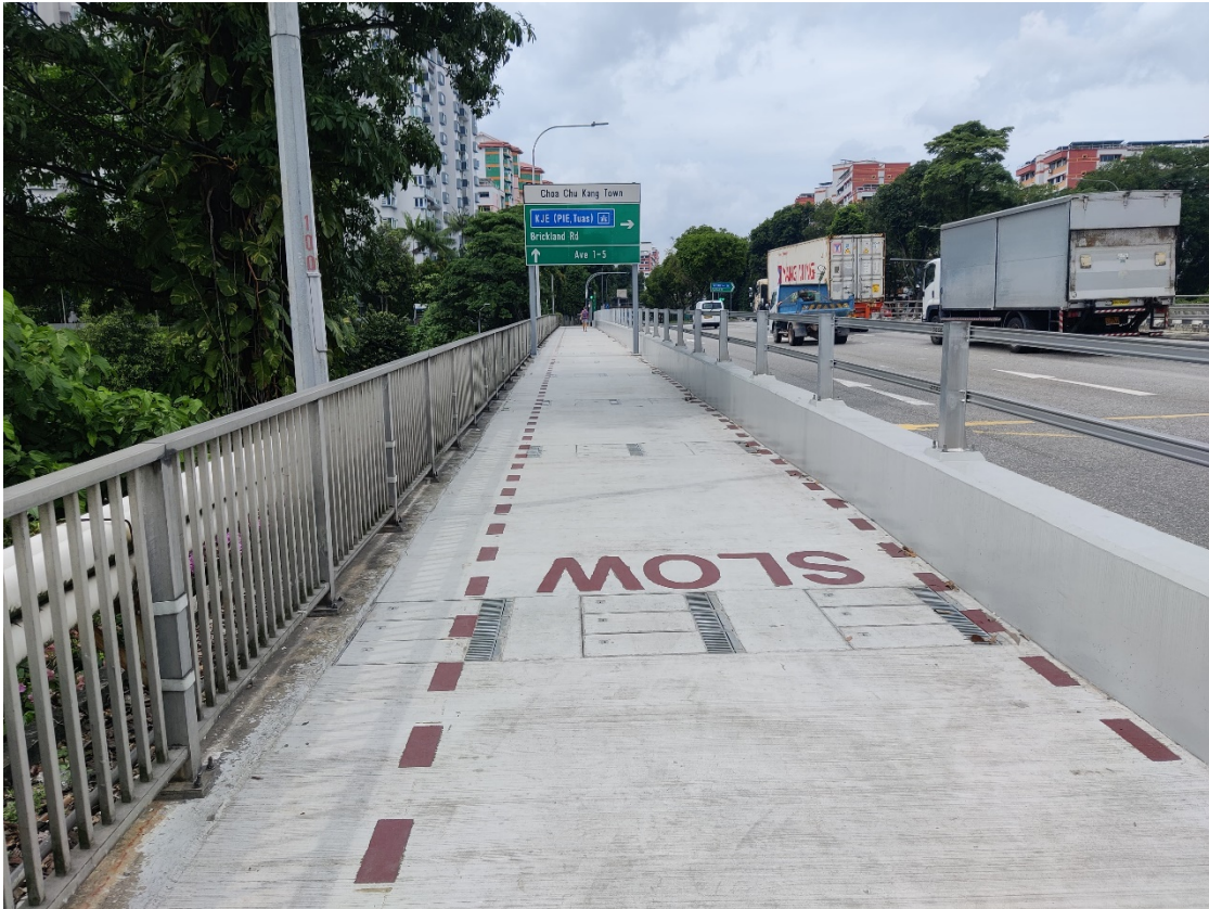
Implemented cycling path along Choa Chu Kang West Flyover by repurposing a segment of the road
