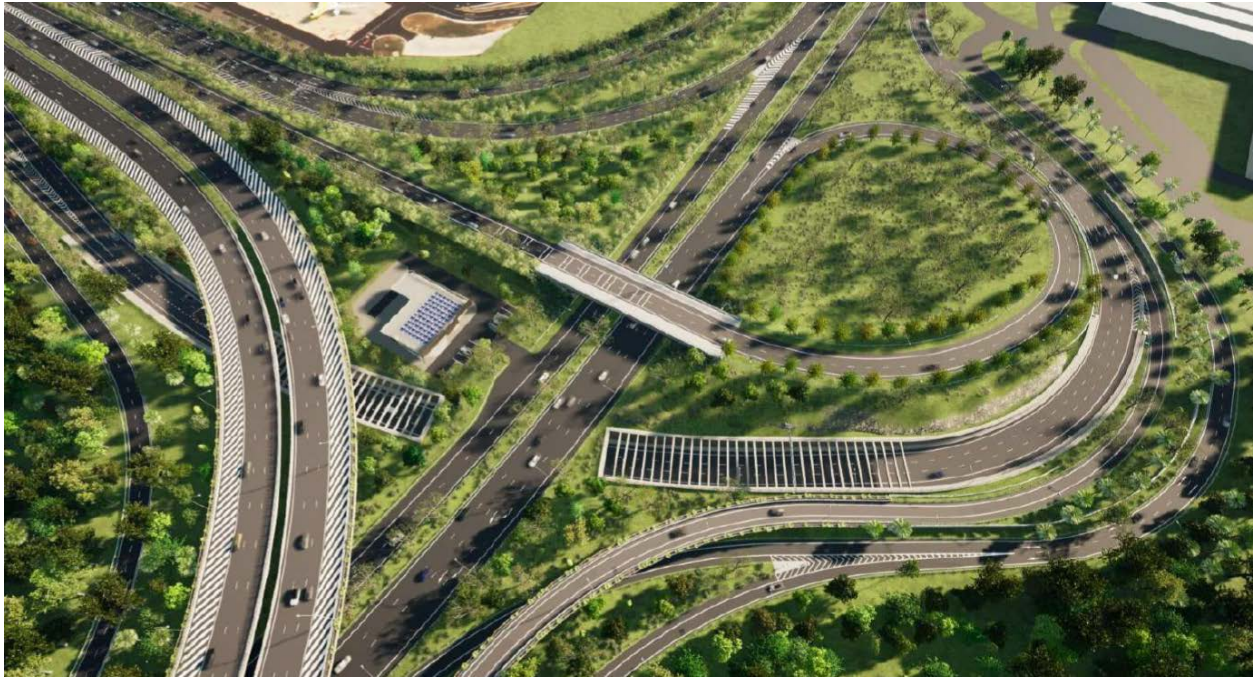
Underpass from Airport Boulevard to PIE(Tuas) and Flyovers connecting PIE to Tanah Merah Coast Road
