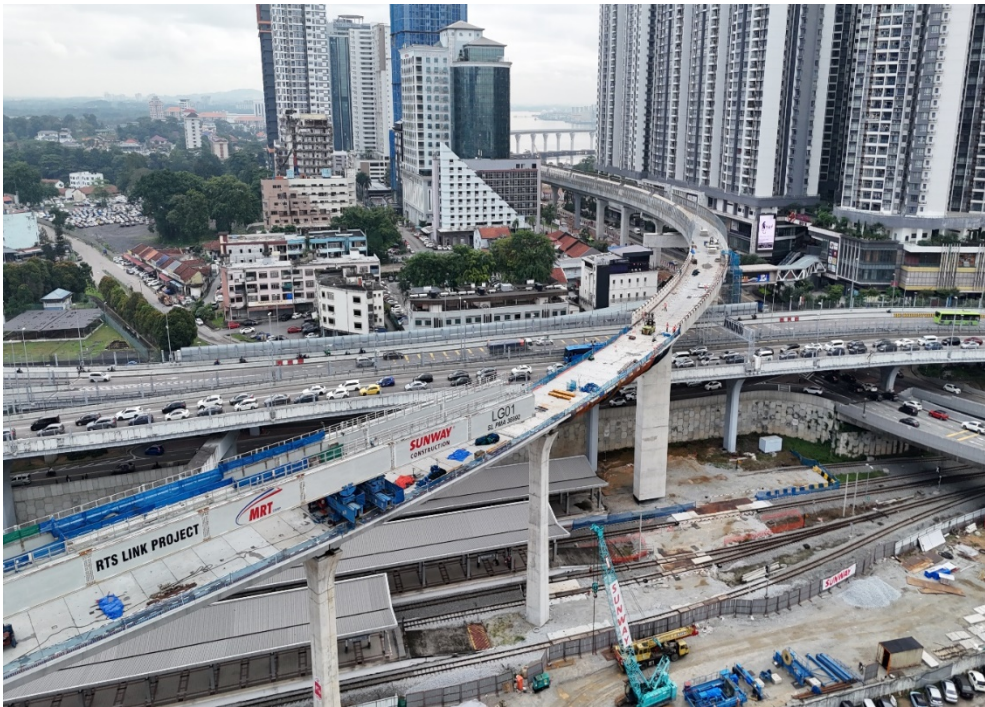
Terrestrial Viaduct along Jalan Tun Abdul Razak
