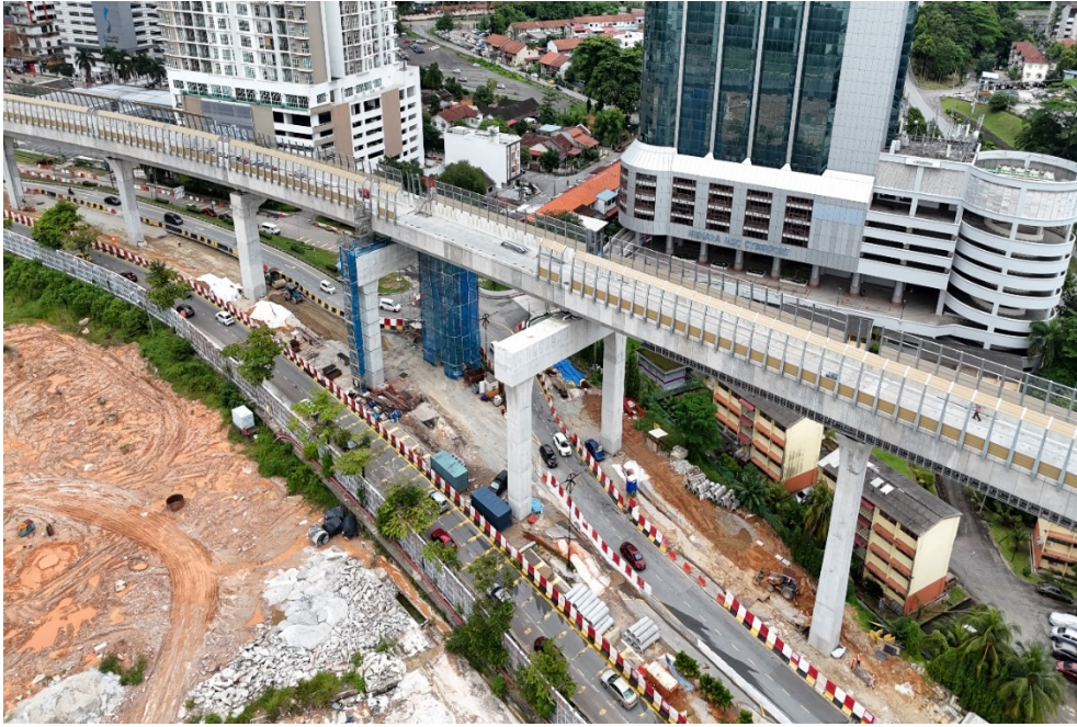
Terrestrial Viaduct along Jalan Ismail Sultan
