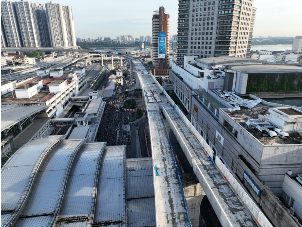
Terrestrial Viaduct along Jalan Tun Abdul Razak
