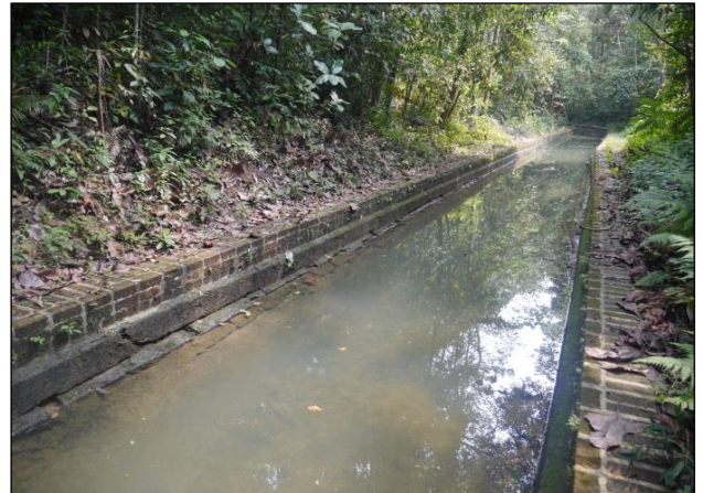
Stream Hd and PUB reservoir interchange waterway
